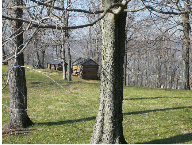
Replica log structures constructed at Fort Duffield
